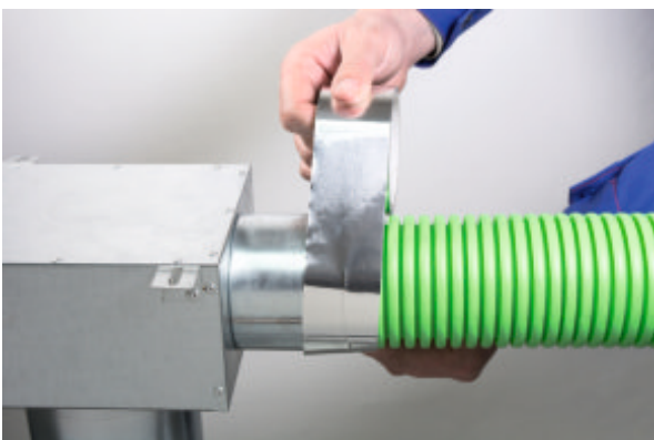
7) Secure the connection using air-tight self-adhesive tape.
